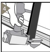
Engage the nailer onto the tongue-side of the board. Drive the nail no further than 1 in (2.5 cm) from each end of the board and 4 to 6 in (10 to 15 cm) from either sides of the center.
