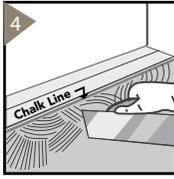
Spread recommended adhesive using notched trowel, from the chalk line/straight edge to approximately the width of two boards. Never spread more adhesive than can be covered in 30 minutes.
